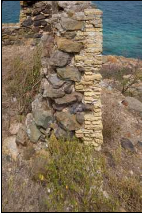
Figure 1 - Brick and Stone Masonry Detail from the Kitchen/Latrine Building
