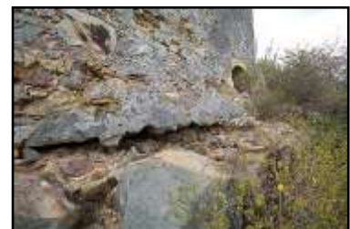
Figure 3 - Degraded/Missing Foundation Detail
