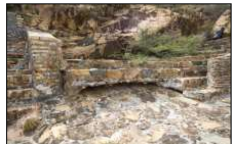
Figure 8 - Terreplein Stairs with Missing Foundation
