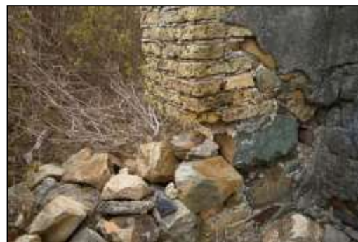
Figure 4 - Missing Masonry from North Pier
