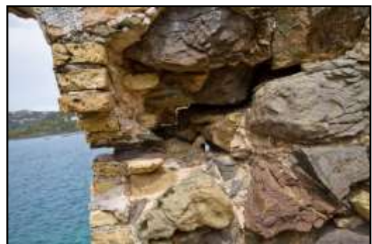
Figure 5 - Missing Masonry at Southern Window
